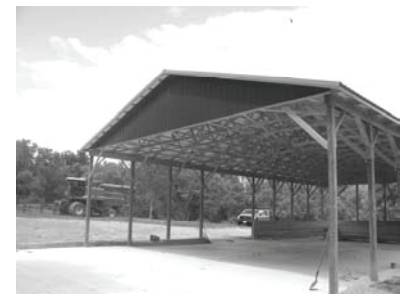
Manure Storage Facility and Heavy Use Area
