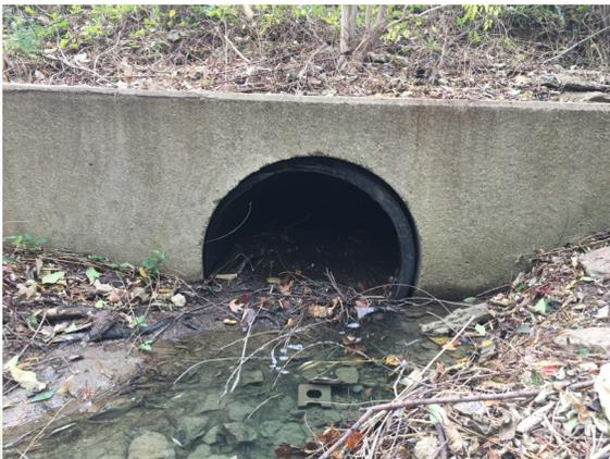
Retention pond outlet structure partially blocked by debris
