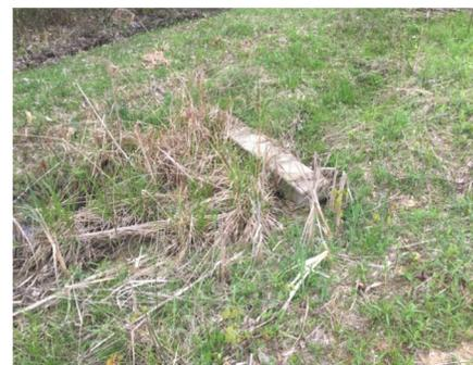
**Blocked inlet to retention pond - Regular cleaning will prolong the life of the structure.**
