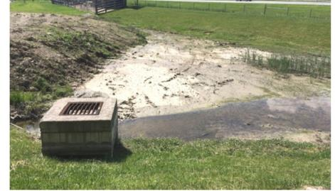
**Excessive sedimentation in a drained basin**
