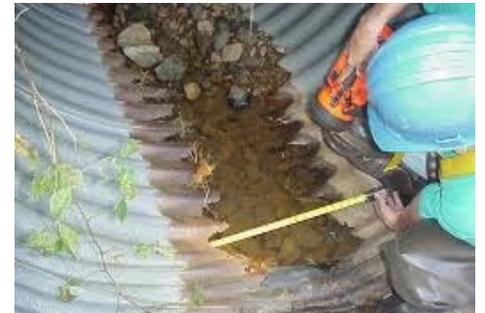
Badly corroded outlet pipe
