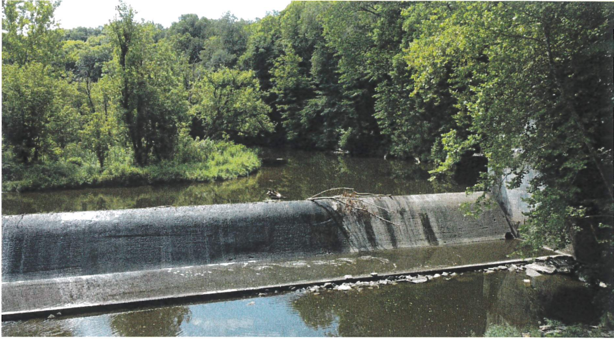
Figure 4. Picture of the dam looking upstream
