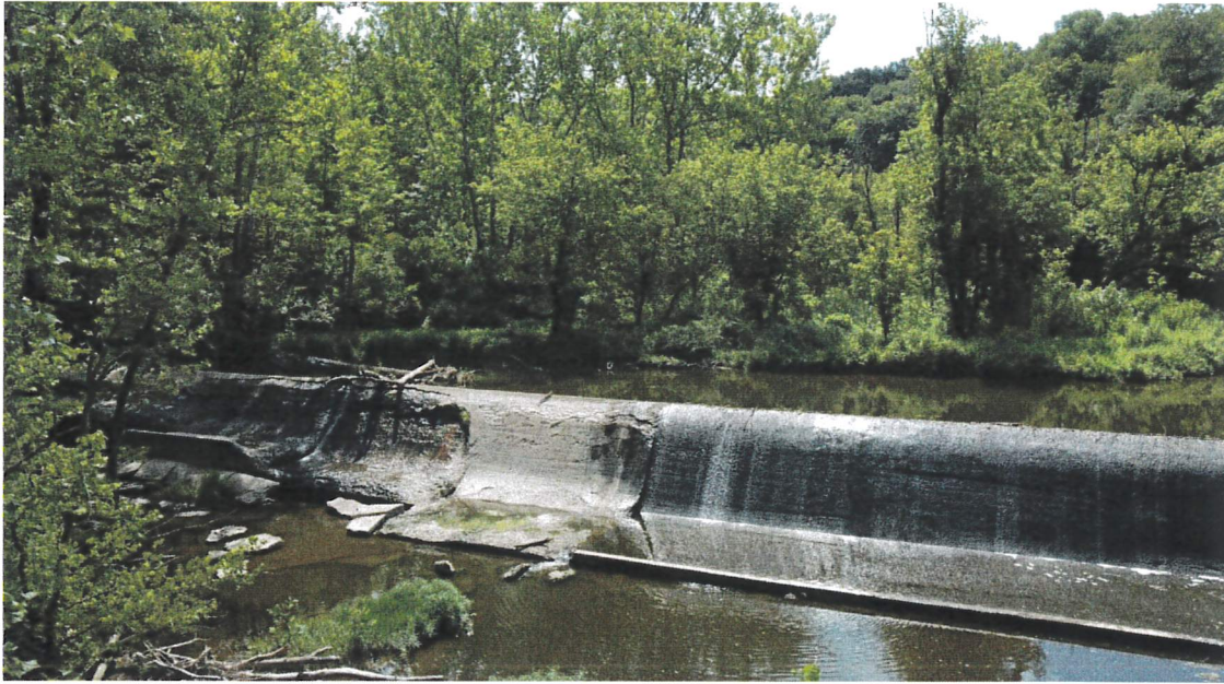
Figure 6. Picture of the dam looking upstream toward the right descending bank
