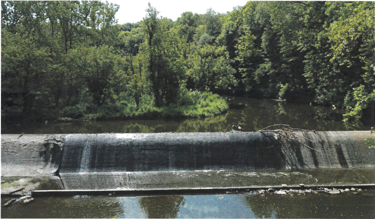
Figure 5. Picture of the dam looking upstream
